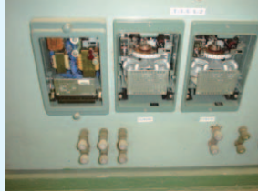
Deterioration of internal parts of protective relays
