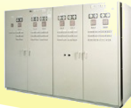
Medium-voltage Distribution Panels
