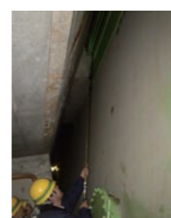
Spraying in a high position (extension rod used)
